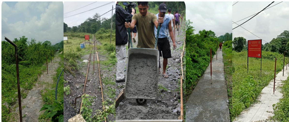
Figure 41: Installation of Electric Fencing as mitigation measures to reduce HEC
