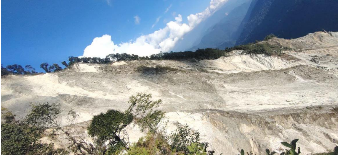
Figure 58: Landslides at Chhudzom
